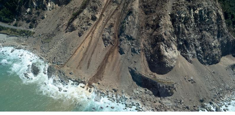
Figure 4: SH1 access along the South Island coast severed by large landslides following the 2016 Kaikoura Earthquake. Similar landslides of this magnitude are expected to occur in Wellington should a major earthquake occur in the region. (Source: Walter Rushbrook / Aurecon)
